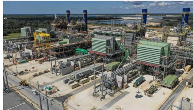
Combined Cycle Gas Turbine station, Florida
