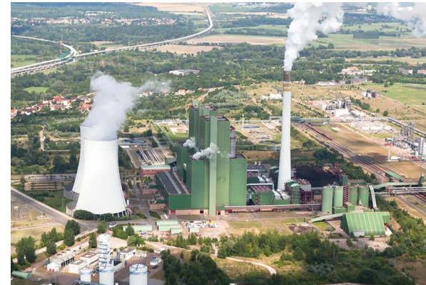
Schkopau Lignite-fired Plant, Germany
